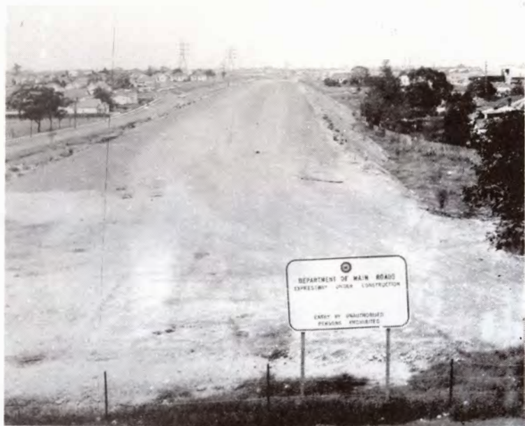
Western Expressway under construction.
