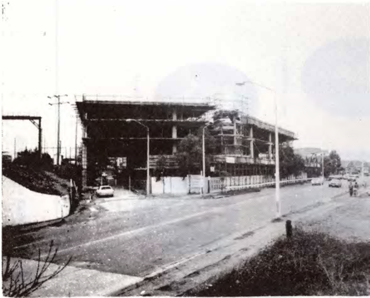
Carparking Station - Bridge Street, Lidcombe.
