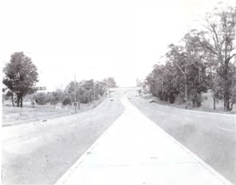
Completed roadworks - Joseph Street.
