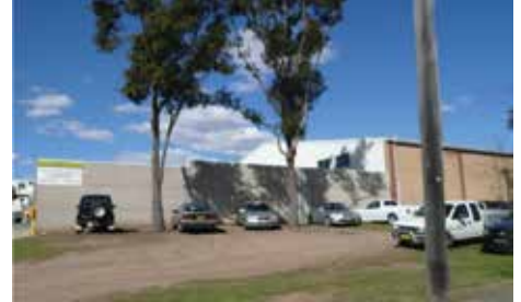
Figure 2: Poor example of blank wall treatment
