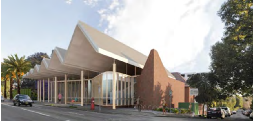
Figure 6.5: Mirvac Design, Proposed library from the corner of Marrickville Road and Lilydale Street, JBA Planning
