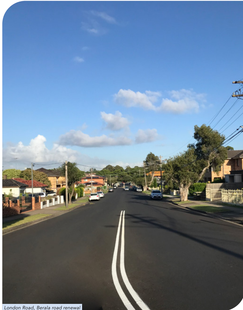
London Road, Berala road renewal
