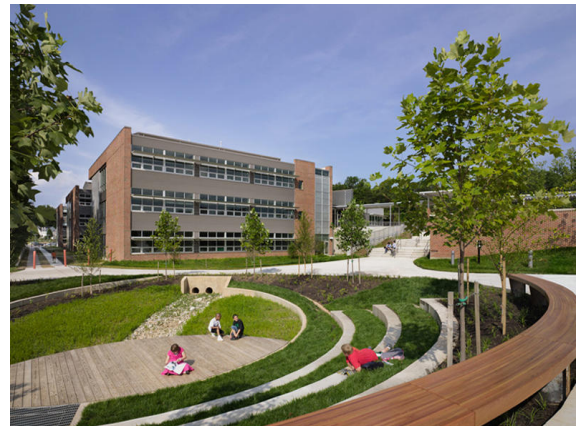
Figure 20 - Bioswale amphitheatre, Manassas Park Elementary School, Virginia, USA. (Source: americainstituteofarchitects.com/top10projects )
