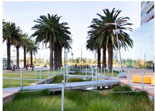
Figure 22 - Melbourne Docklands - Overland flow path as a passive recreational space. (Source: www.aecom.com.au )
