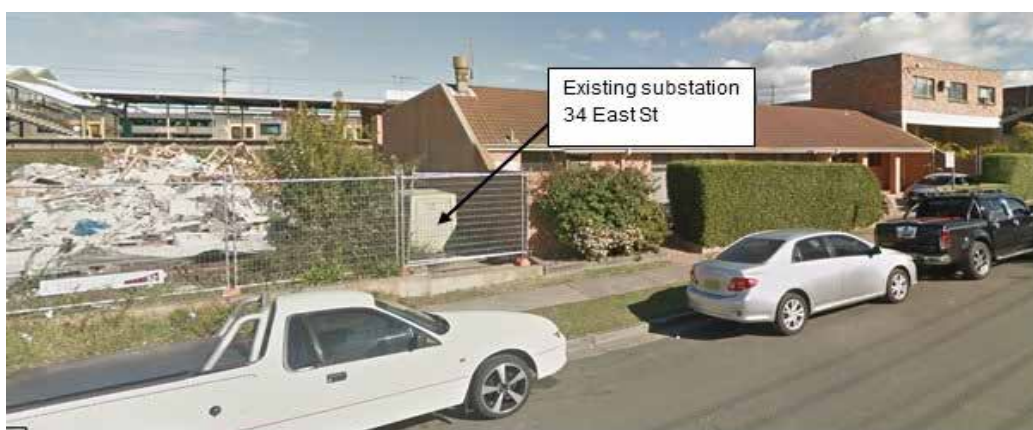
Figure 4.3.7.2.4 Existing padmount substation at 38 East Street, Granville
