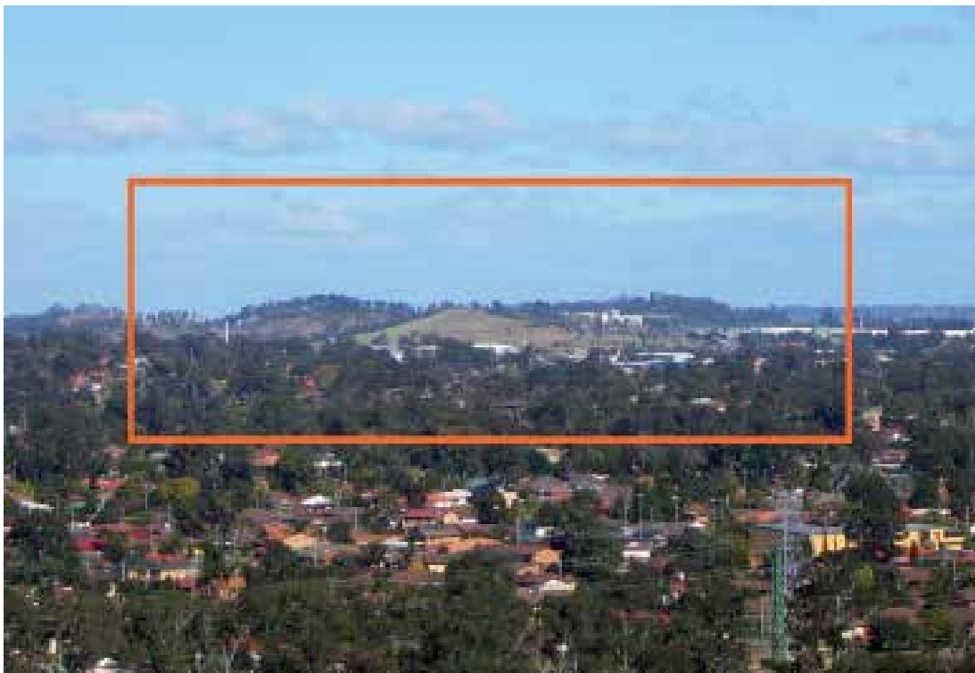
Figure A2.2.1 Looking South West towards Prospect Hill, Buckleys Road, Winston Hills
