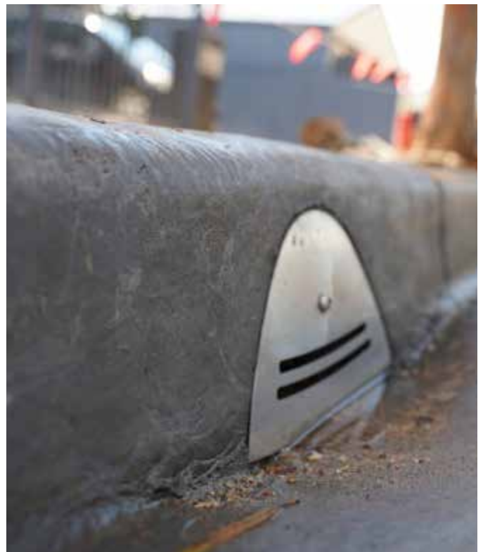
Tree inlets passively water trees by directing stormwater into the tree pit (Photo courtesy of spacedownunder.com.au)
