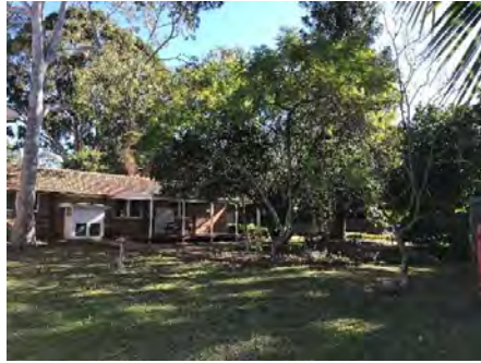
Figure 25: Northern addition to the house, facing north-west (Source: NBRARCHITECTURE)
