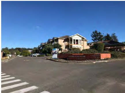
Figure 15: View of the entrance to Cardinal Gilroy Village (Source: NBRARCHITECTURE)
