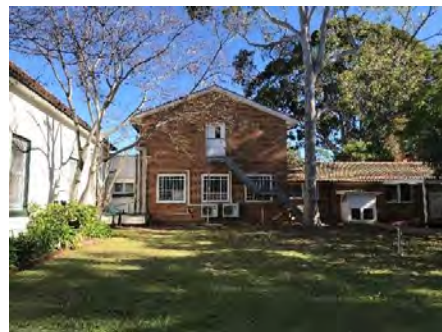
Figure 24: Eastern façade of the northern wing to the house (Source: NBR SARCHITECTURE)
