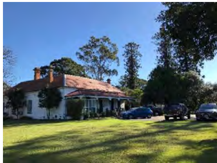
Figure 21: South-east corner of the house, viewed from the lawn (Source: NBR SARCHITECTURE)
