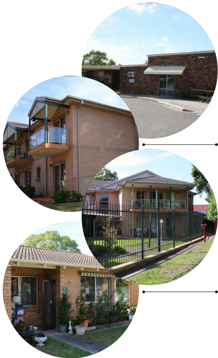
View of Community Centre Building
