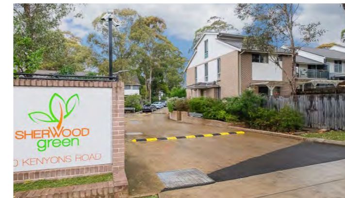
11 Sherwood Green Entrance from Kenyons Rd
