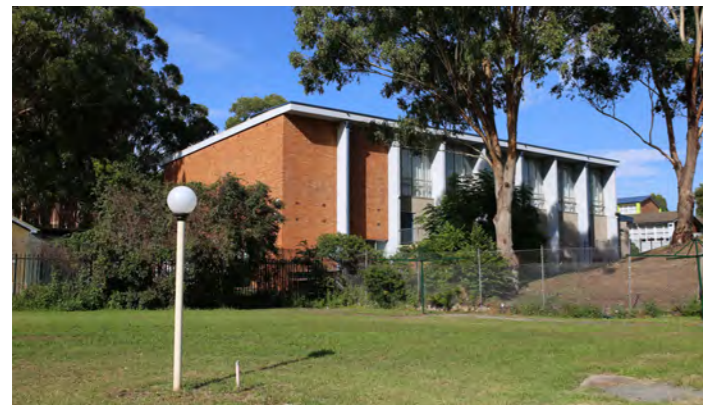
21 View of Cerdon College building from south-west corner of site
