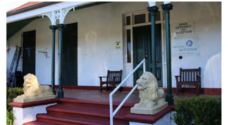
32 Heritage Building Verandah
