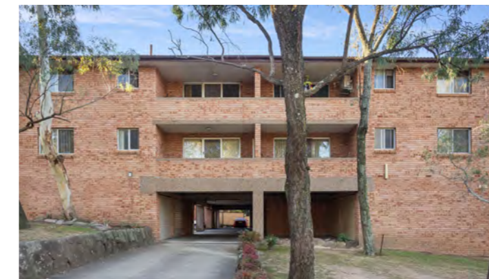
25 Apartment building on Torrens Street
