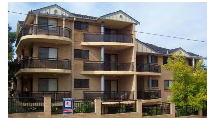
26 Apartment building on Torrens Street
