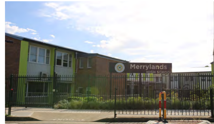
22 Merrylands High School from Bristol Street
