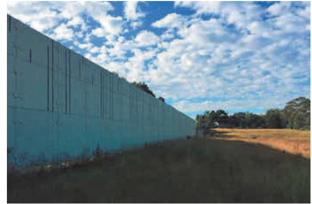
2. VIEW OF THE WALL CROSSING THE Site
