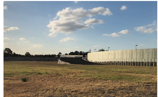
6. VIEW OF THE ELEVATED PLATFORM
