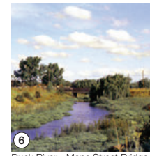
6 Duck River - Mona Street Bridge
