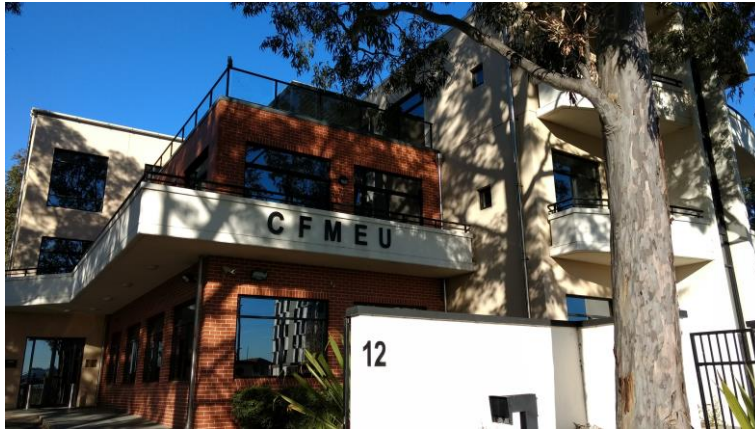
Figure 3: 10-12 Railway Street - comprising of a 3-storey office building
