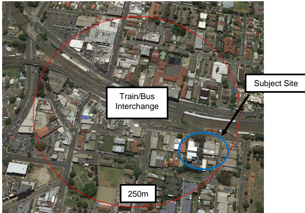
Figure 1: Lidcombe train station walking catchment (subject site highlighted with blue boundary)
