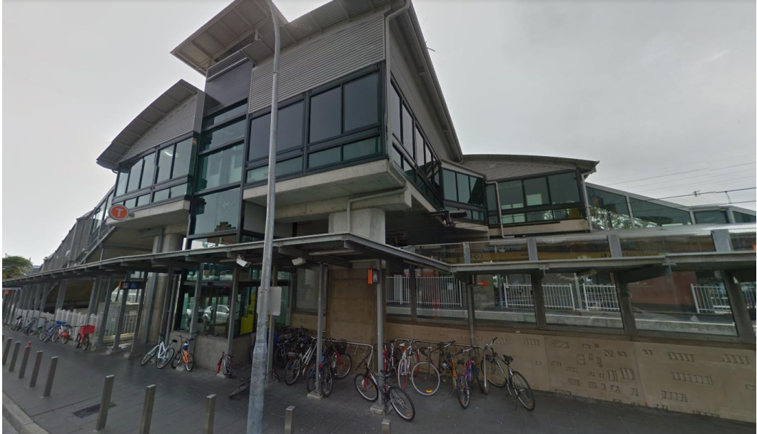
Figure 8: To the north - Lidcombe Train Station
