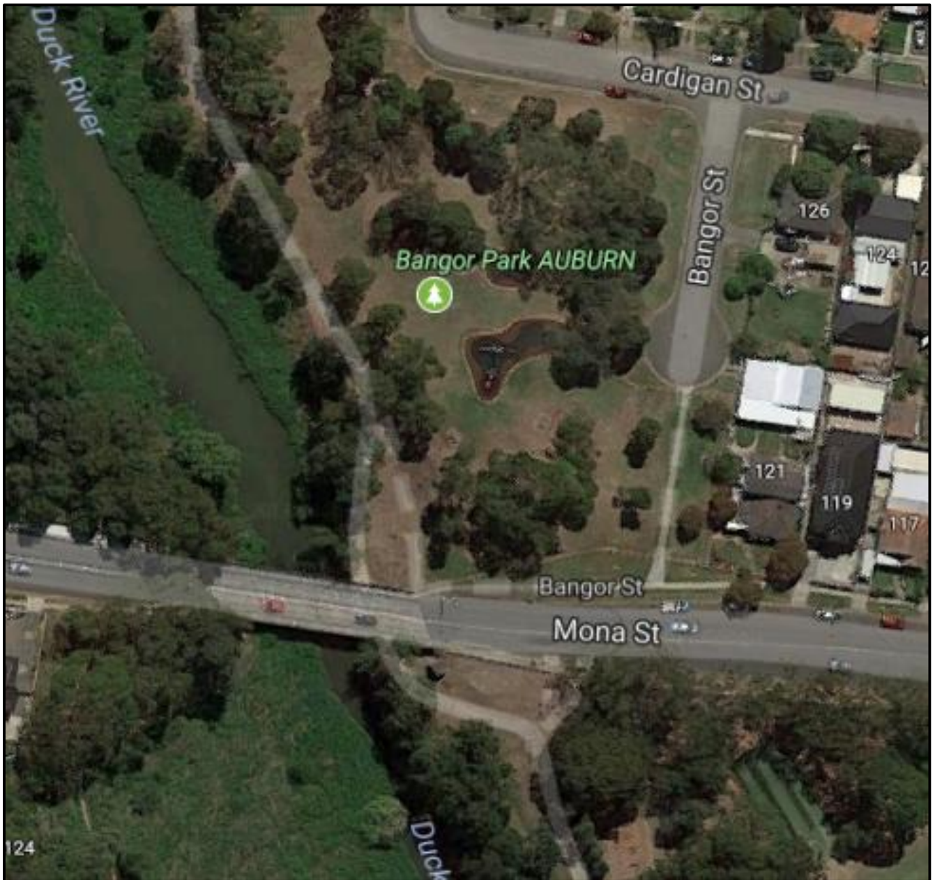
Figure 4.12 : Mona Street Bridge
