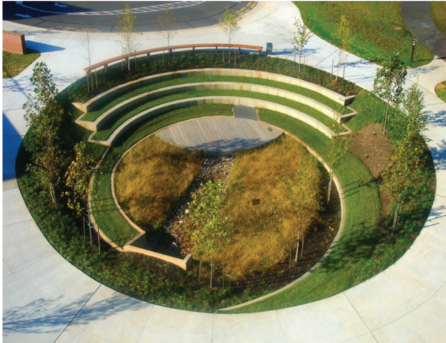
Figure 5 - Bioswale amphitheatre, Manassas Park Elementary School, Virginia, USA. (Source: americaninstituteofarchitects.com/top10projects )
