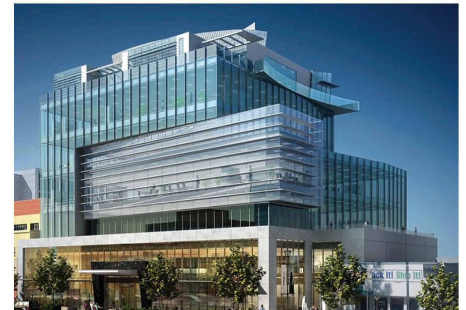
Figure 46 - The horizontal and vertical architectural elements provide interest and break the monotony of the elevation and scale of the building
