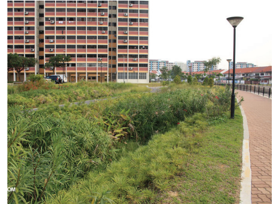
Figure 7 - Bioswale - Singapore, a green link. (Source: www.aecom.com.au )
