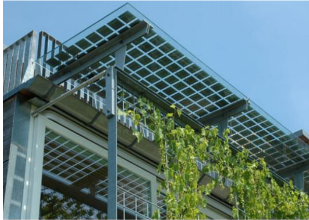
Figure 7: Integrated PV in shading structure
