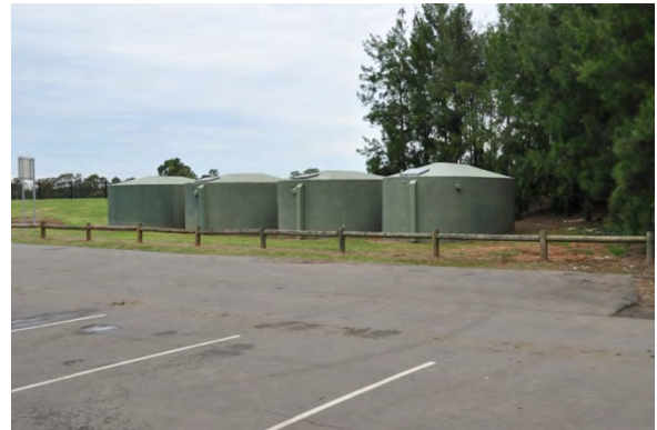
Figure 13 Above ground reuse storage tanks in Jack Ferguson Park
