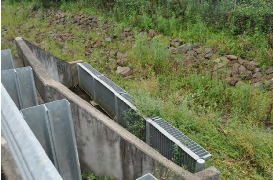
Figure 20: WQD055 Transitway Trash Rack
