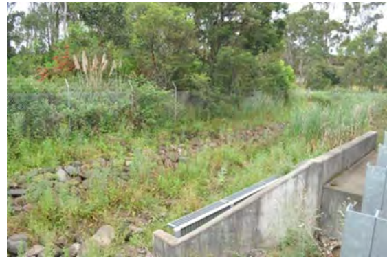
Figure 9 Culvert beneath LPT and upstream embankment across Munro Creek
