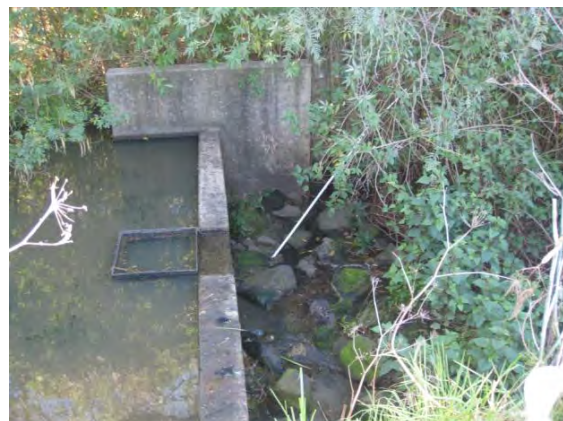
Figure 10 Jack Ferguson Pond Outlet Weir Control
