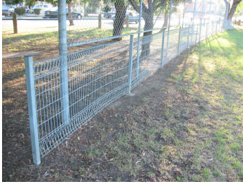
Fence constructed by Council to protect adjoining homes and streets from damage by cricket / footballs.
