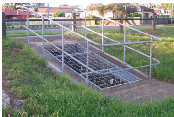
Major surcharge facility located on Burnett Street adjacent to swimming centre
