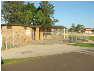
Southern amenities building.
