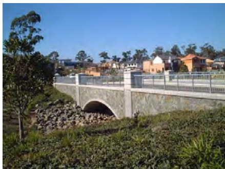
Naoi Bridge across Driftway Reserve
