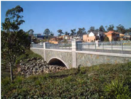
Naoui Bridge across Driftway Reserve
