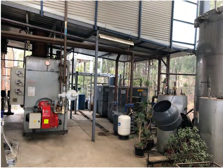
Exterior of laundromat building – boiler area.
