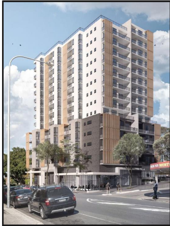
View from Station Street in the north-east
