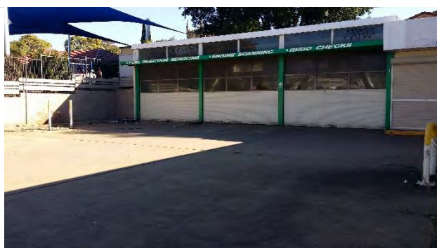
Photograph 2: The former mechanic workshop annexed to the service station at the eastern section of the site.
