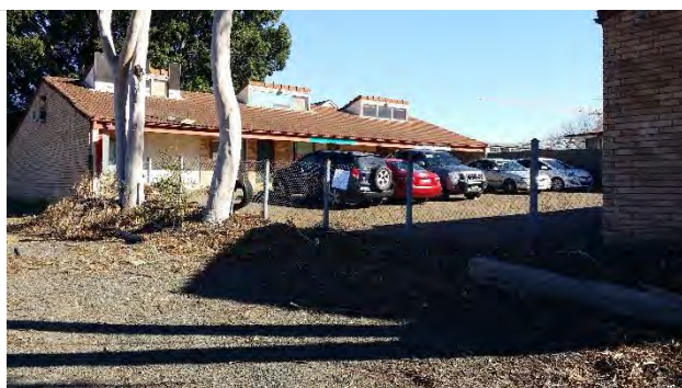
Photograph 4: The commercial buildings and the carpark in the western section of the site.
