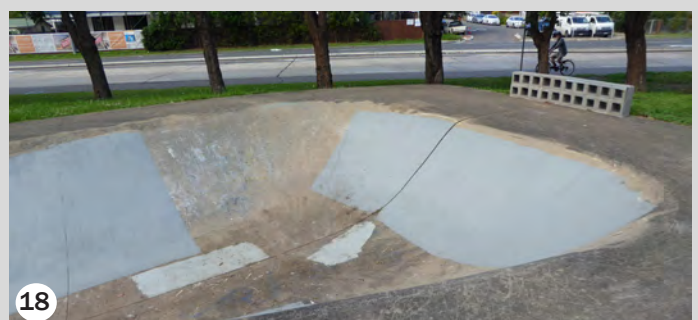
Plate 2: Condition of existing facilities
