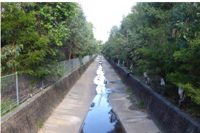
Plate 3: Haslams Creek canal
