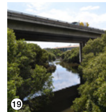
19 M4 Western Motorway - Duck River, Clyde
