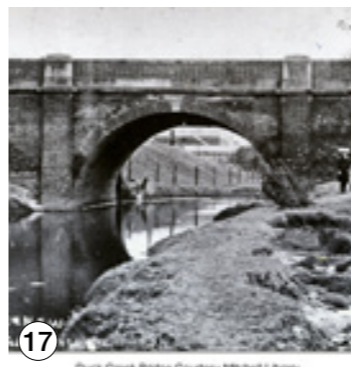
17 Duck River Bridge at Clyde - 1833-1836
