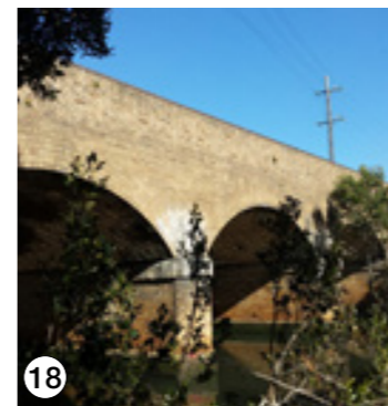
18 Duck River Bridge at Clyde
