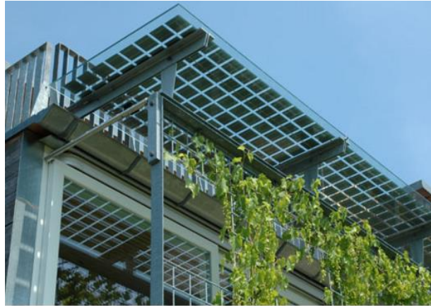
Figure 7: Integrated PV in shading structure
