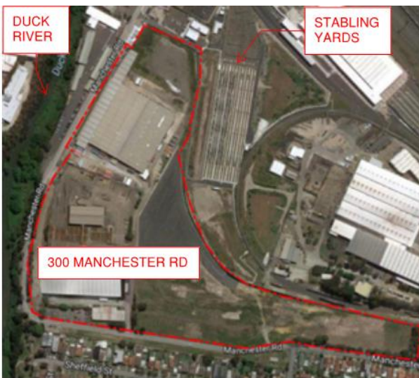
Figure 1 Existing Site Conditions
