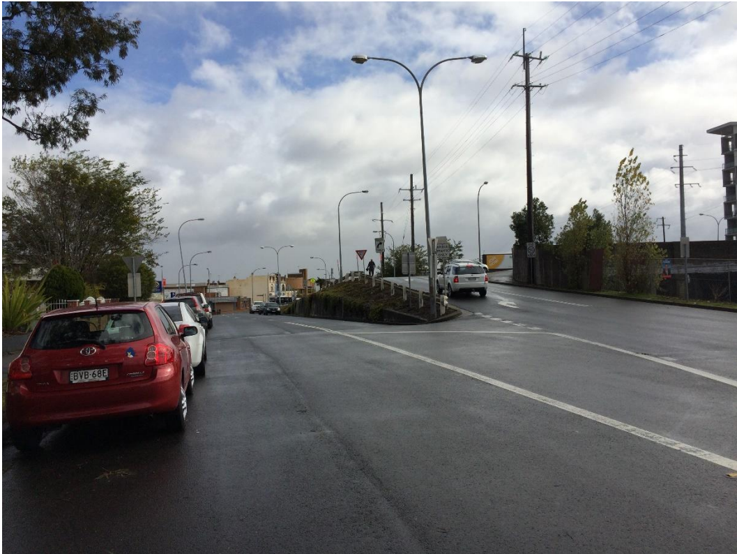
View looking west along Railway Street from the northern frontage of the site
