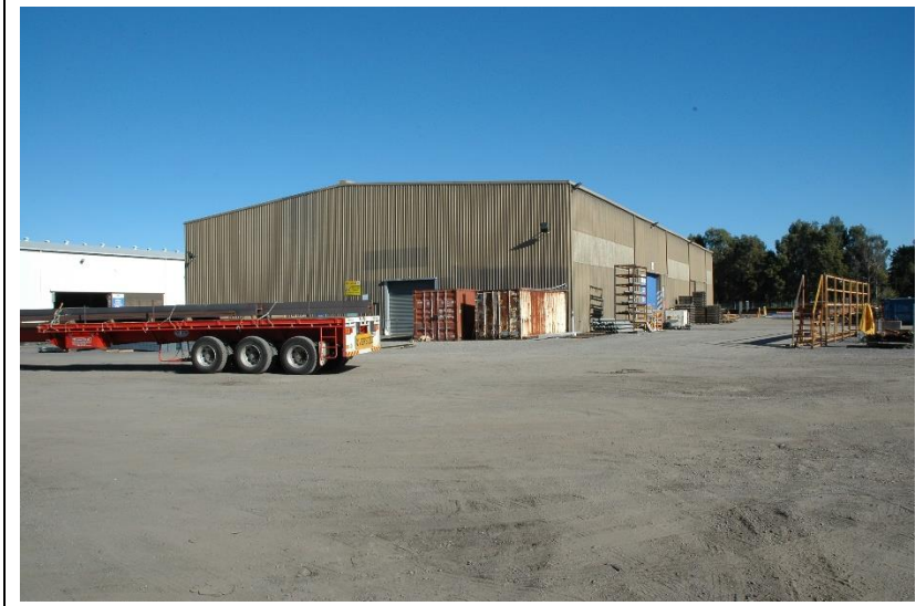
Figure 10: Warehouse in Lot 11.
