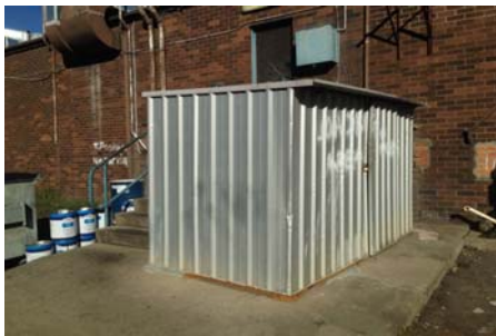
View of rear of property showing chemical storage shed Looking west. Inspected on 27.03.2015
