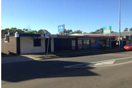
View of 108 Station Street, Wentworthville frontage Looking southeast. Inspected on 27.03.2015
