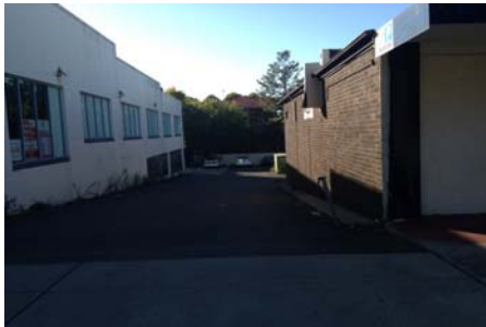
View of asphalt sealed driveway to rear carpark Looking east. Inspected on 27.03.2015
