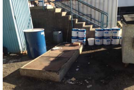
View of rear of property showing grease pit and chemical /oil storage area. Looking north. Inspected on 27.03.2015
