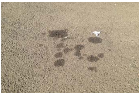
View of carpark showing typical stains on surfaces Inspected on 27.03.2015
