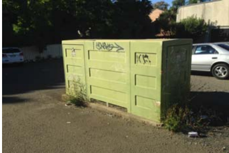
View of carpark showing high voltage electrical transformer box. Looking southeast. Inspected on 27.03.2015
