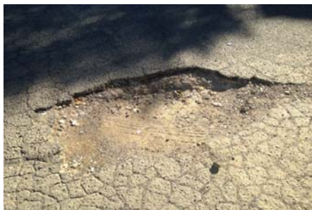
View of carpark showing cracks and holes within surfaces. Inspected on 24.03.2015
