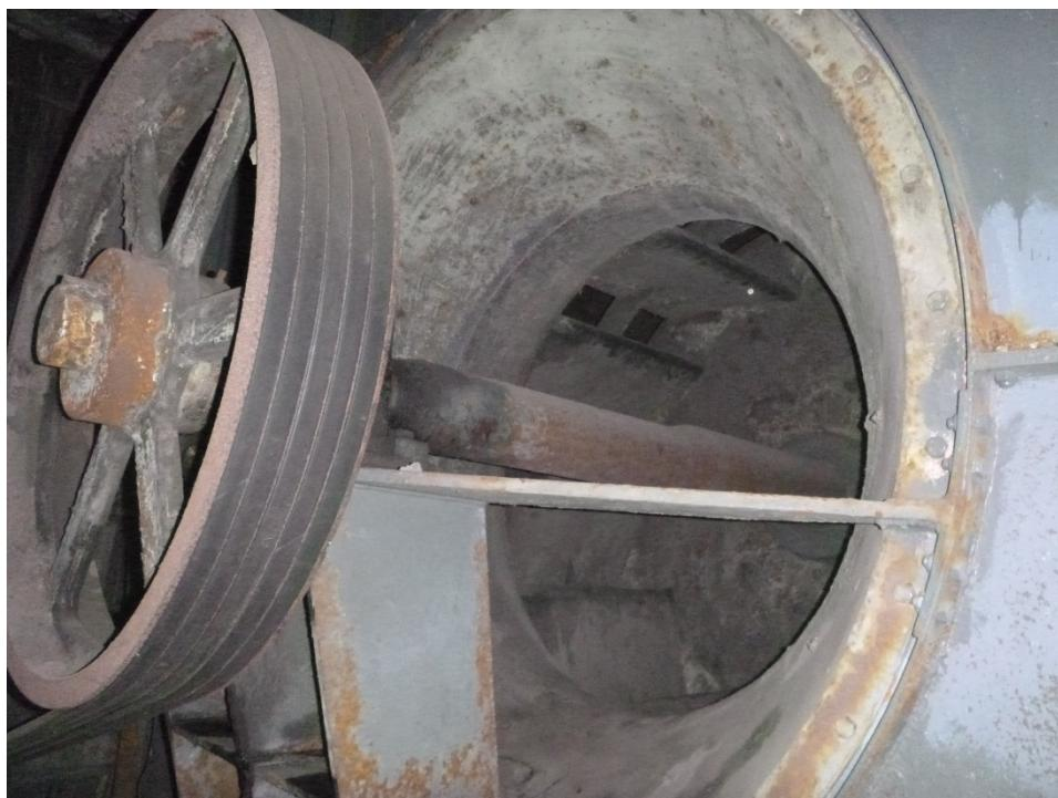
**Photo 9: Belt turn wheel in a room of the central area of Building 3.** The wheel diameter would be approximately 2 m in diameter, and the shaft would be 3 – 5 m long (difficult to see the back as the room was very dark). Ellie was unsure what it was used for or if it is still operational.
