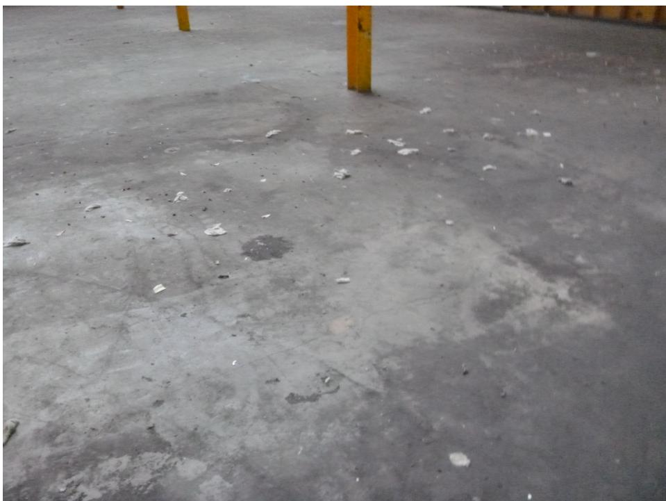
**Photo 12:** Staining and debris on the floor of Building 3.
