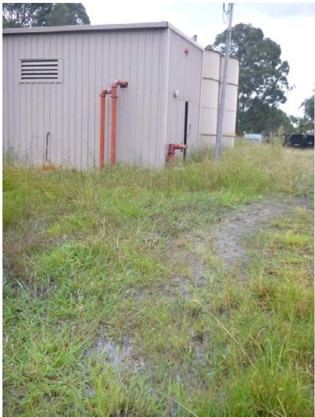
**Photo 29:** The pump house and the water tank, located west of building 1. The tank was leaking at the time of inspection (as shown by the wet grass area in the foreground) and apparently it had been leaking over the three days prior.
