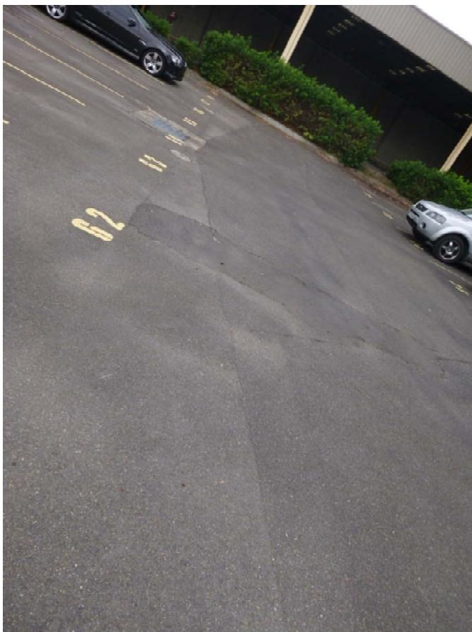
**Photo 31:** The ground surface in the central car park showing numerous saw cuts, potentially for the installation of a drainage system.
