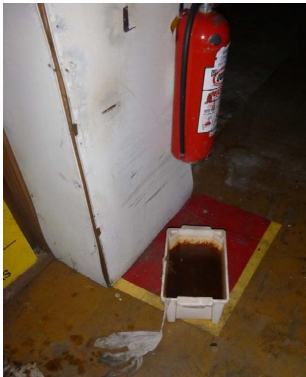
**Photo 18:** tub collecting water leaking from the roof. Ellie thought that the colour was from rust in the roof.
