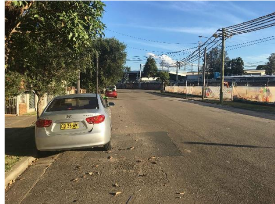
Figure 2.7: St Hilliers Road (looking south)
