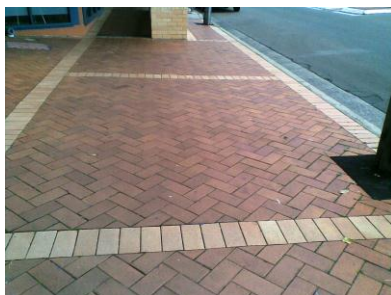
Red Brick Paving - medium-good condition
