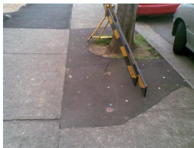
Concrete - poor condition
