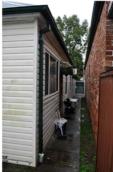
18. East wall. Vinyl siding.
