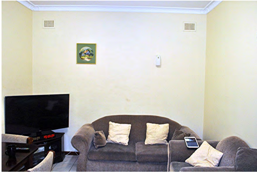
23. Lounge Room- plasterboard wall and ceiling linings.
