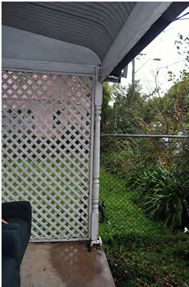
17. Turned post, lattice.
