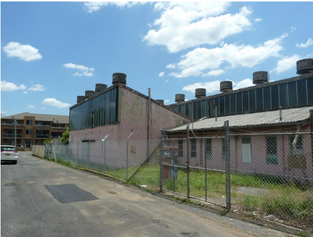
Figure 5 Rear of the commercial warehouse building at 12 William Street, viewed from the access lane
