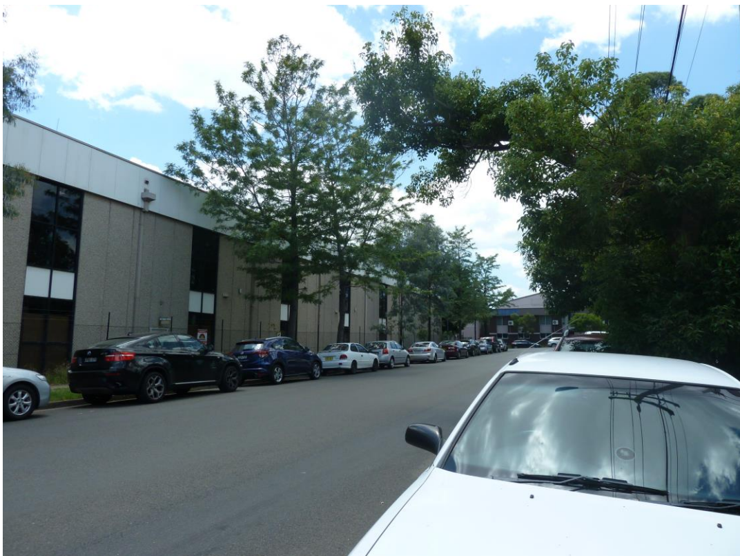
Figure 12 Industrial building at 1 Memorial Avenue, to the north of the site
