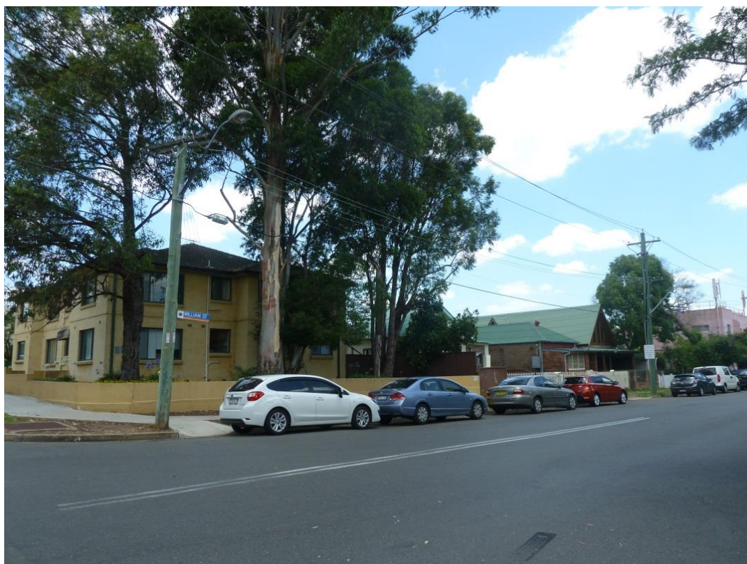
Figure 7 Residential flat building at 2 William Street, viewed from William Street
