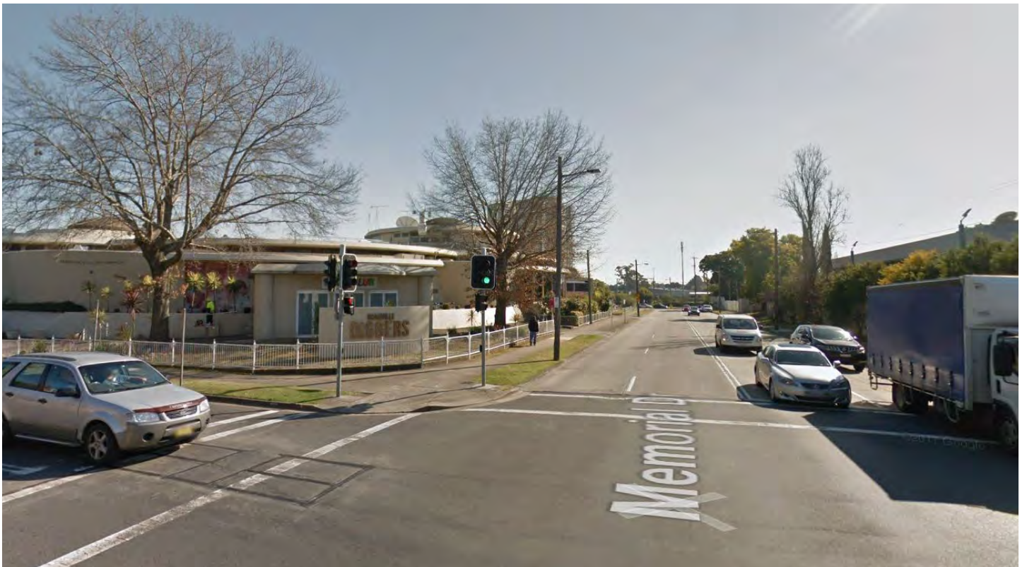
Granville Diggers Club with view to the new higher density development at Granville, Town Centre in the distance. (Source: Google Streetview)
