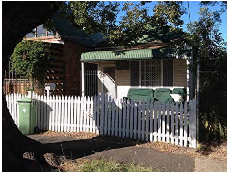
Figure 20 – 10 William Street, heritage item Source: Archinex
