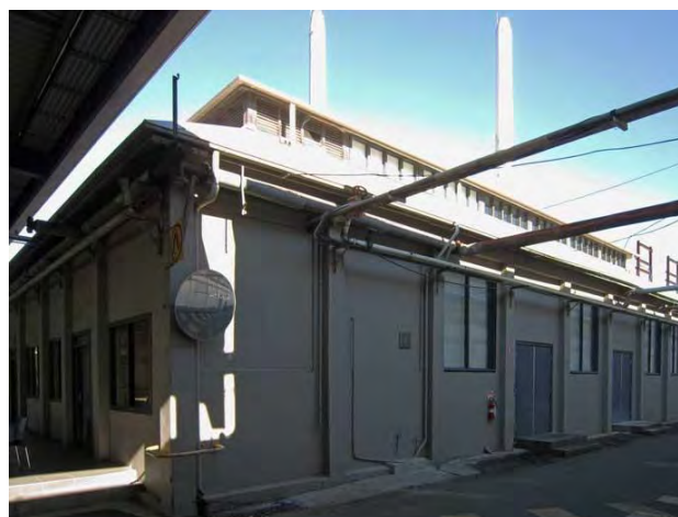
Figure 85 The exterior of the John Austin Centre, showing the early louvre panels in the clerestory. (Source: Orwell & Peter Phillips Architects)
