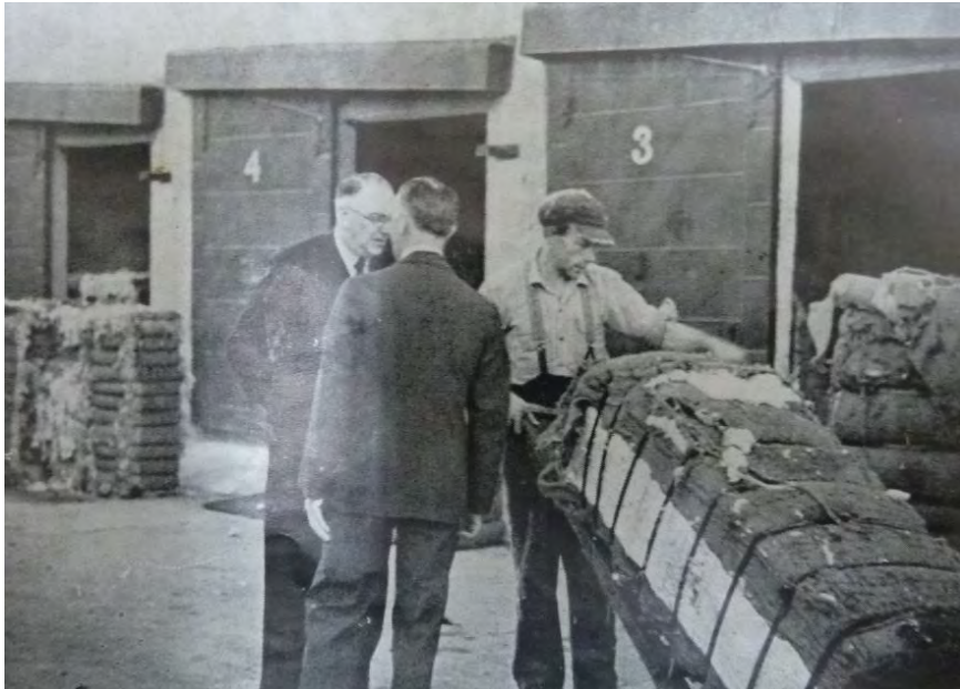
Figure 37 Bond's Industries Ltd General Manager W Hermon Slade (left) inspecting a bale of cotton arriving at the Cotton Bale Stores, originally a row of seven concrete fire-proof bunkers with counterweighted steel sliding doors. The bales, weighing up to 4-500 lbs, are bound with metal hoops. (Source: Pacific Brands archives)
