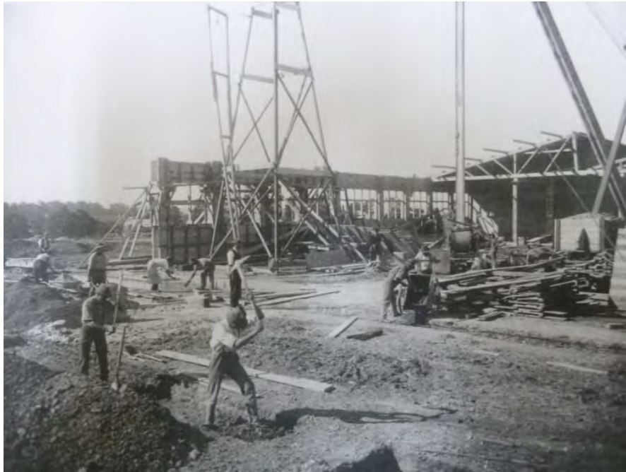
Figure 5 'Lathing in the foundations for the cotton spinning mill, Wentworthville' circa 1923. (Source: Pacific Brands archives)
