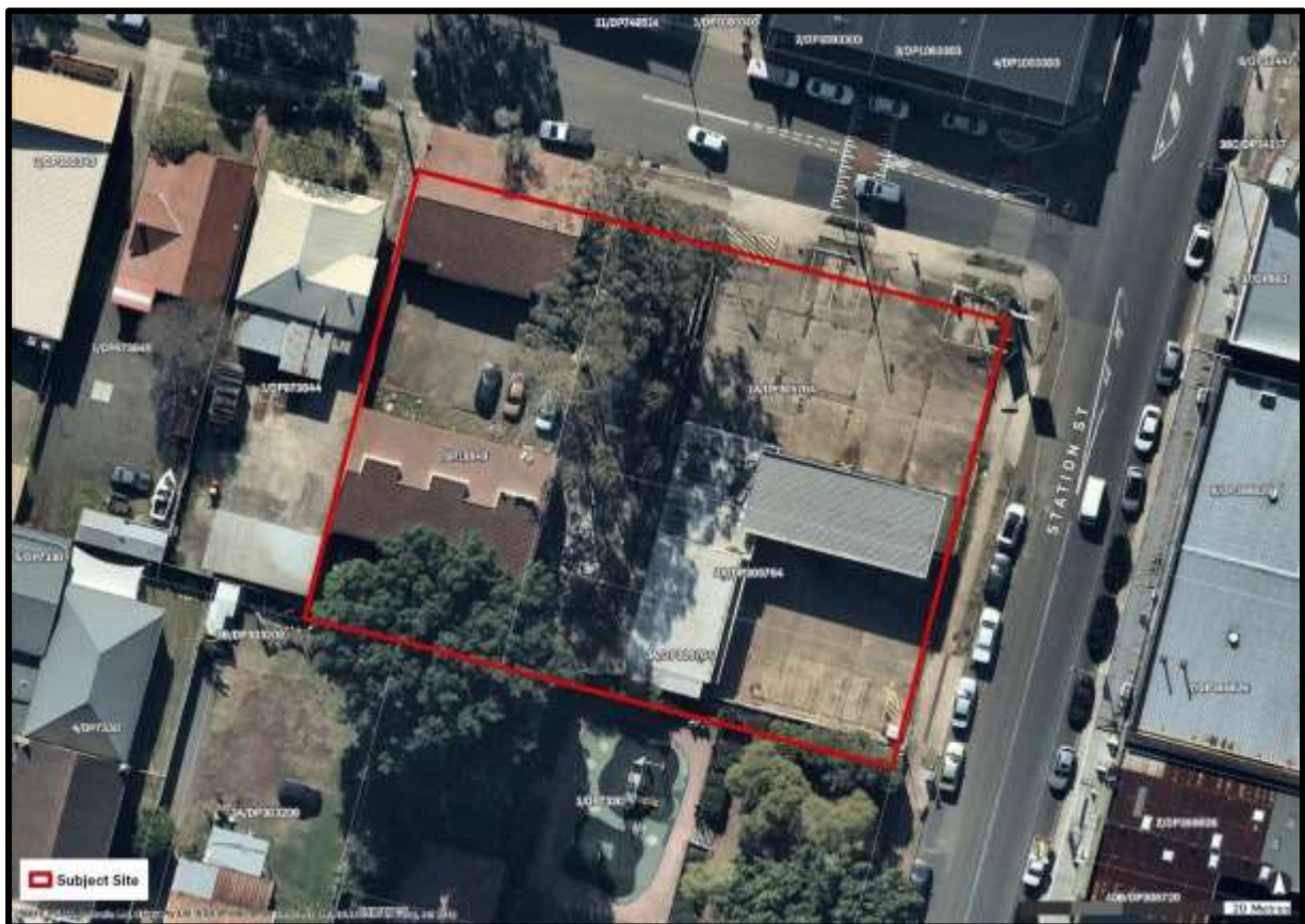
Figure 2 – Aerial view of the site (outlined in red)
