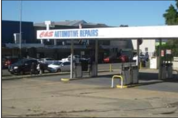
Former service station, as viewed from Pritchard Street East
