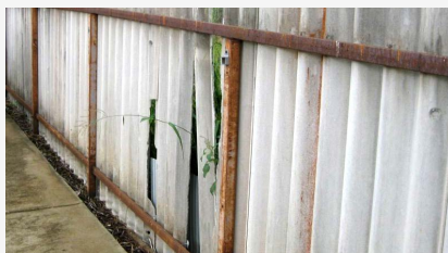
Asbestos fencing in need of repair*
