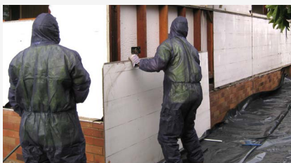
Safe asbestos removal in progress*
