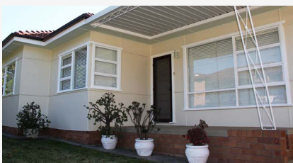
Classic fibro home with asbestos cladding/eaves
