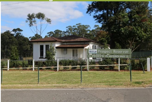
Entrance to Prospect Reservoir.
