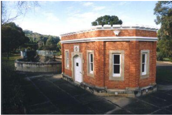
Lower Valve House and Receiving Basin on the Lower Canal (Source: NSW Office of Environment and Heritage, State Heritage Register listing sheet for Prospect Reservoir)
