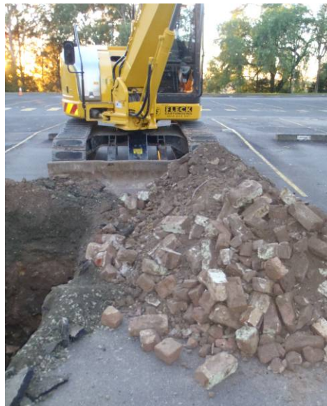
Photo 3 – Rubble at TP40
