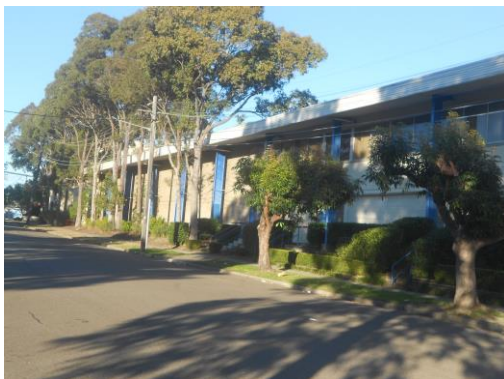
Figure 4 - View of existing building from Percy St
