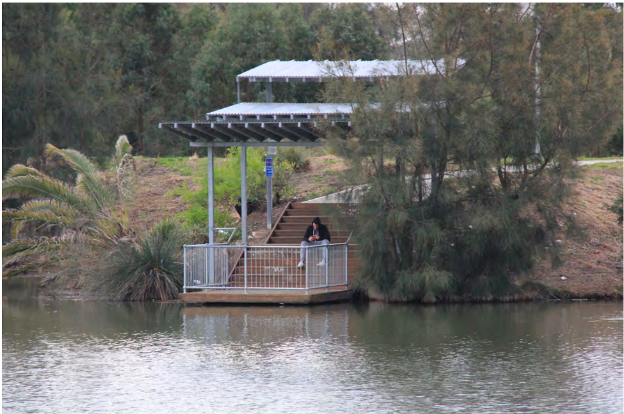
Shelter deck to northern dam wall
