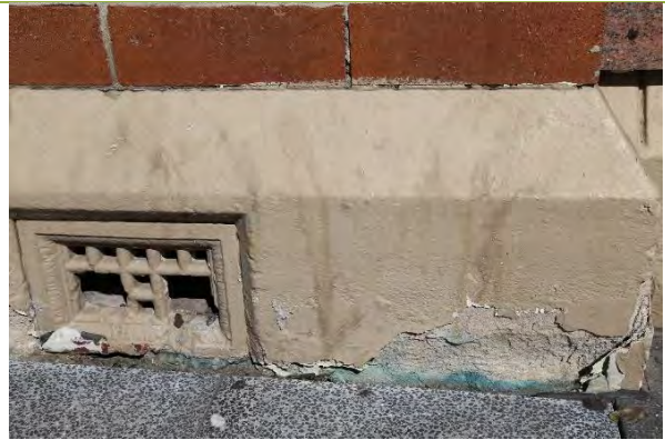
Detail to damage caused to sandstone footings by acrylic paint. Not also damage to vent.
