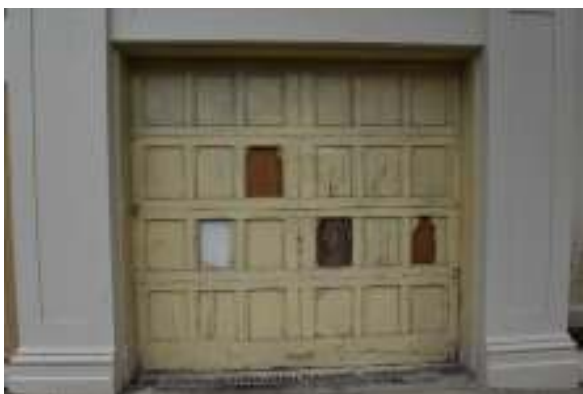
View of modified garage entry along the eastern elevation. Highly dilapidated timber garage door.
