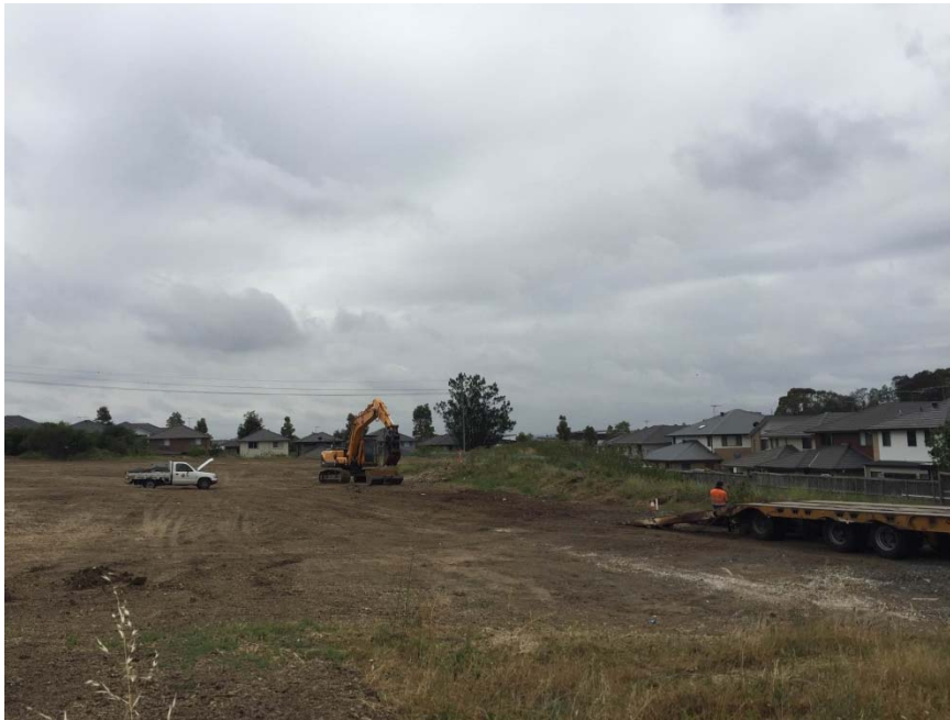
Figure 2: Existing site looking North East
