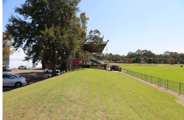
View east to main grandstand at Melita Stadium.
