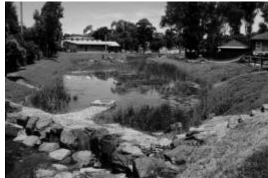
View of the reconstructed Pendle Hill Creek with turfed banks and macrophyte planting.
