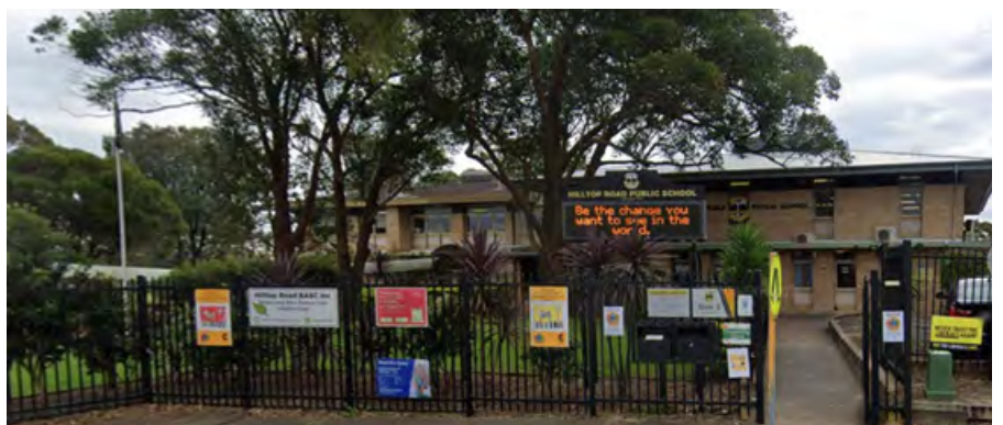
Figure 27 Hilltop Road Public School (Source: Google Maps)
