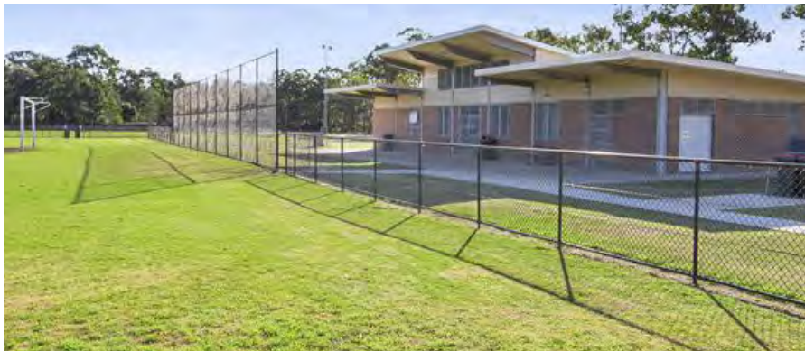
Figure 265 Progress Park (Source: Cumberland City Council)
