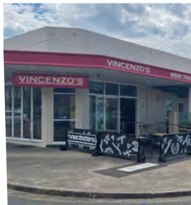
Figure 98 Refurbished Corner Italian Restaurant Building
