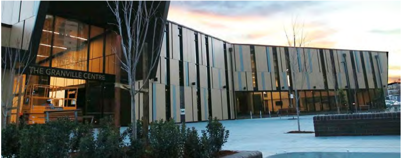
Figure 40 Granville Community Centre (Source: Cumberland City Council)
