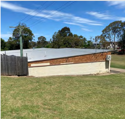
Figure 359 Rear Built form
