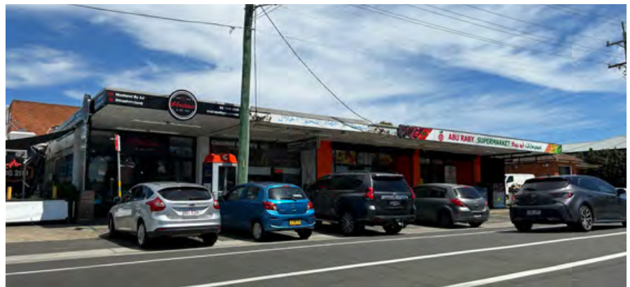
Figure 222 Single Storey Retail Shops
