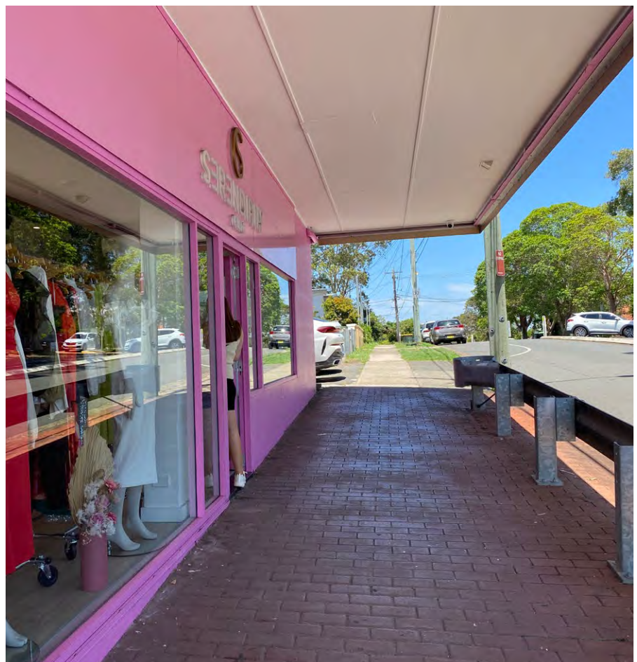
Figure 393 Awnings Providing Shading to the Footpaths
