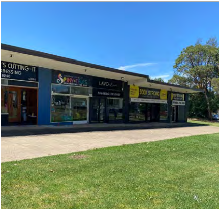
Figure 358 Renovated Awnings and Front Facade
