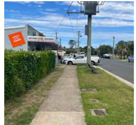
Figure 94 Footpaths along Irrigation Road
