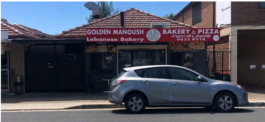
Figure 449 Single Storey Pizza Shop
