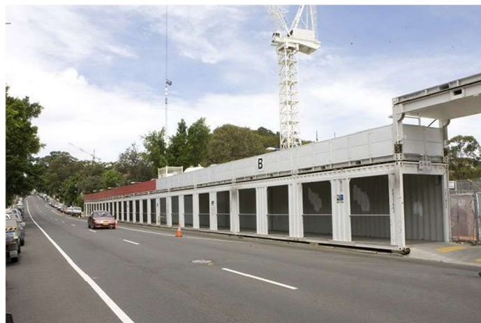
Image – Typical Type B Hoarding
