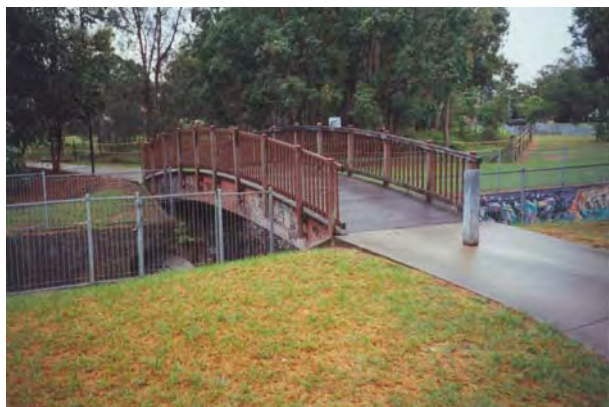
This bridge provides pedestrian / cycle access the concrete channel
